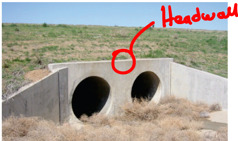
Square edge in headwall – The end of the culvert barrel is flush with the headwall
