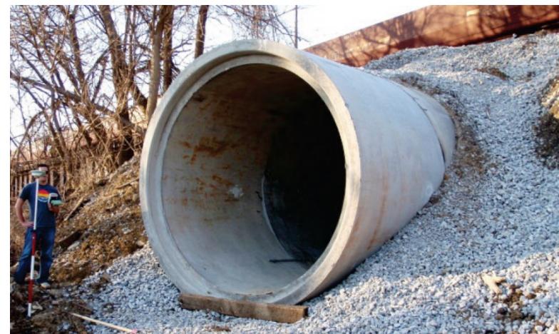
Groove edge projecting – A concrete pipe culvert section extends beyond the fill or headwall. Groove end is a socket end.
