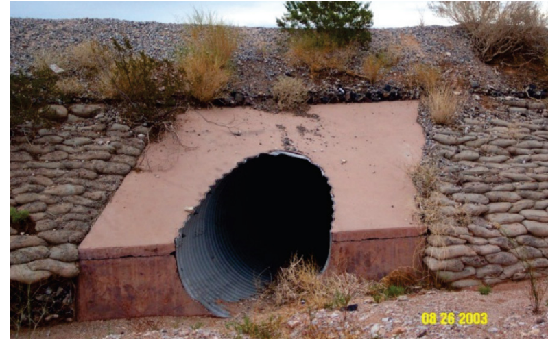
Mitered entrance – The culvert barrel is cut so it is flush with the embankment slope
