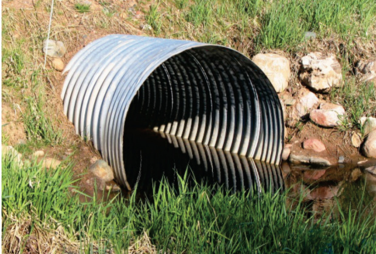
Thin Edge Projecting – The culvert barrel projects out of the embankment
