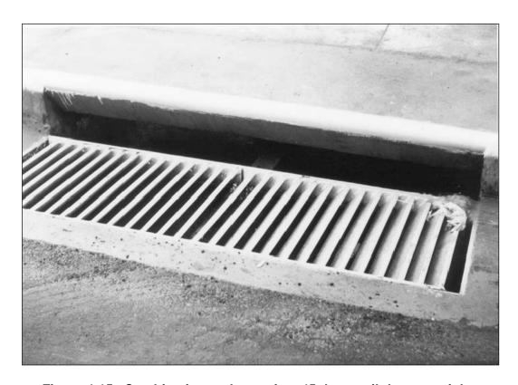
Figure 4-15. Combination curb-opening, 45 degree tilt-bar grate inlet.
