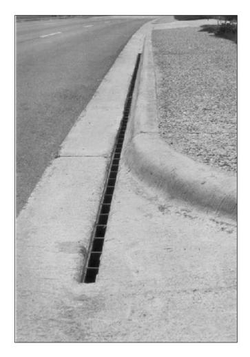
Figure 4-14. Slotted drain inlet at an intersection.
