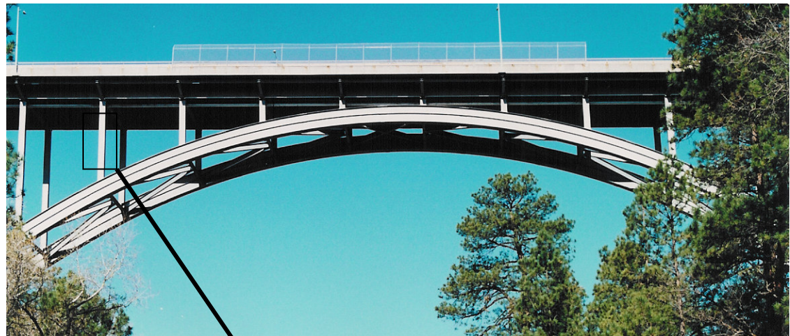
Canyon Bridge, Los Alamos, NM (photo courtesy P.M. Anderson)
